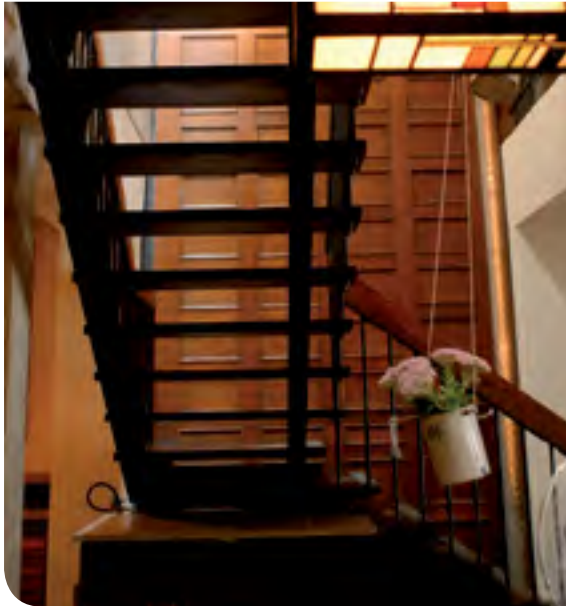
Circulation spaces, including stairs are kept free of clutter and offer good visual access between spaces.
