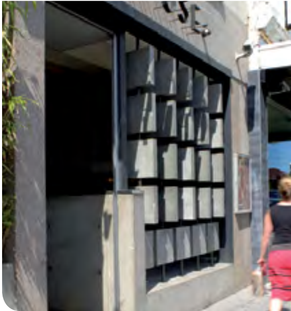
Doors and windows should not allow patrons to spill out onto adjoining public spaces.
